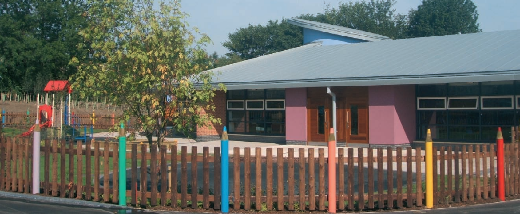
Kings Oak Primary Learning Centre in Barnsley, South Yorkshire, built by Carillion
