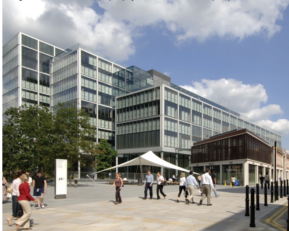
Design and build is now used on complex projects, such as Foster's Bishop's Square
